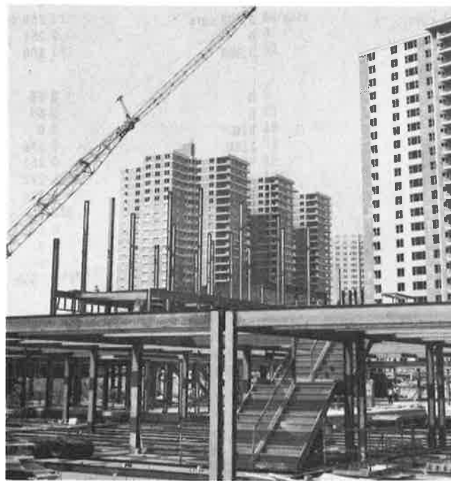
Views of construction at Co-op City, October, 1968
